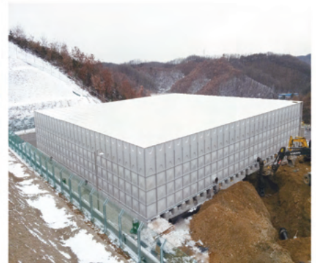
Roof panel assembly
