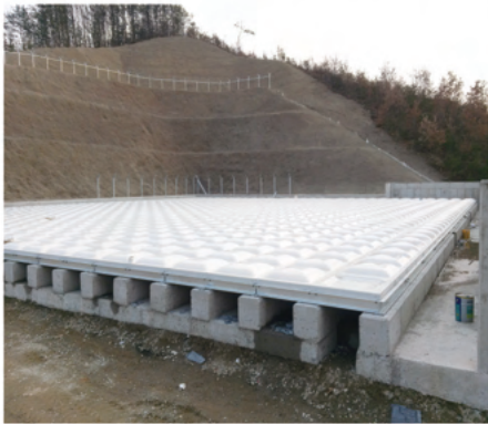
Base concrete PAD & Bottom panel assembly
