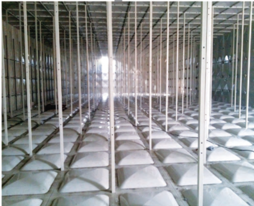
Internal tie-rod & Roof support assembly
